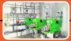
The water then goes through the chemical feed building again where fluoride and phosphate are added for dental health and corrosion control.
