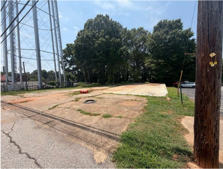
Existing Building Foundation
